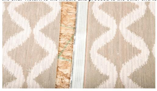
3. Move your iron at an even speed, approximately 3 feet per minute, all the while pressing the carpet into the adhesive behind the iron with your hand or a seam roller (Smooth type, rather than spiked roller). Slide a flat, heavy object along the seam to keep the carpet flat as the tape cools. You must allow for sufficient cooling time before stretching.
